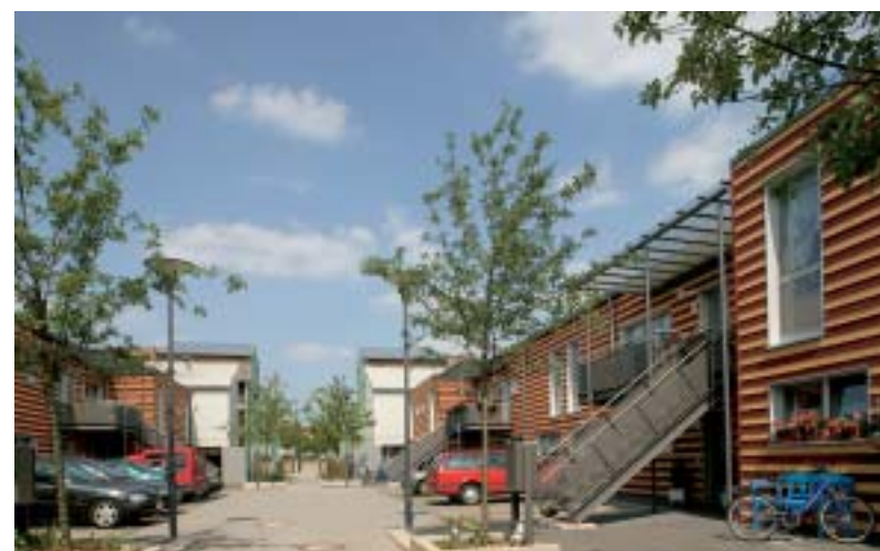
INNENHOF – SOLARCITY SOLARCITY – INNER COURT
